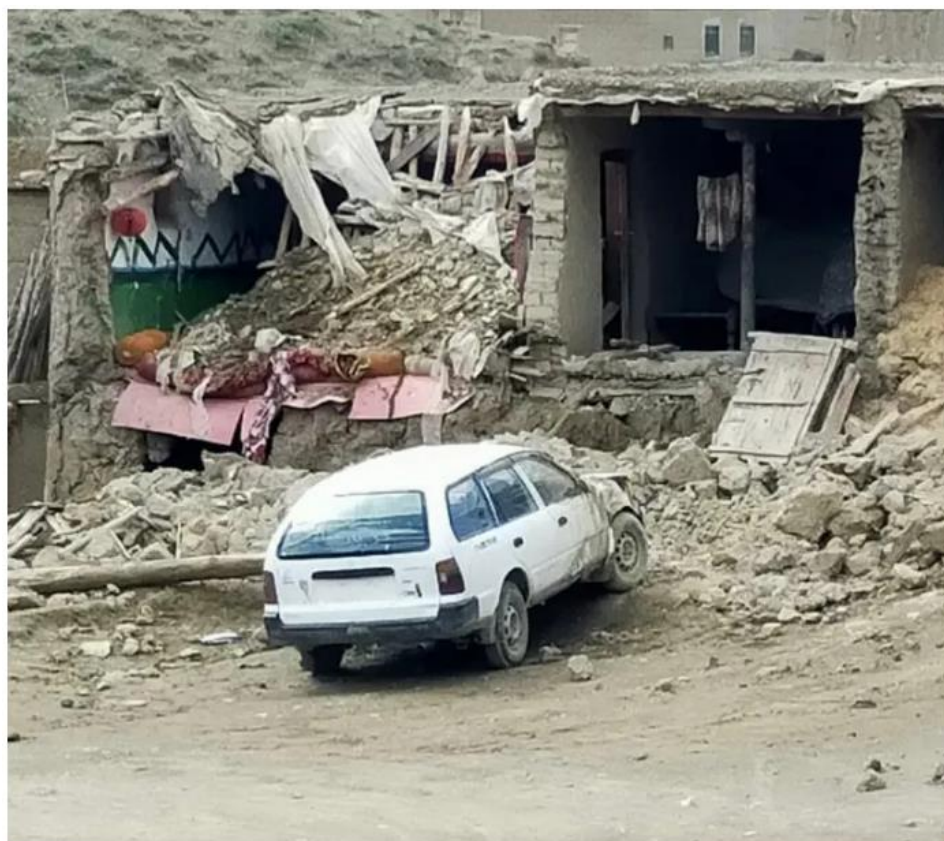
Homes were razed to the ground by a 5.9 magnitude earthquake [Al Jazeera/Stringer]
